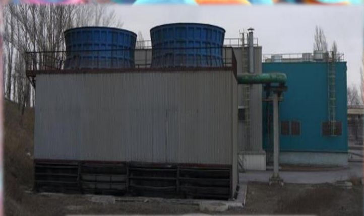
Algae and legionella in cooling towers
