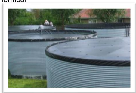
Fixed cover stretched over a water silo
