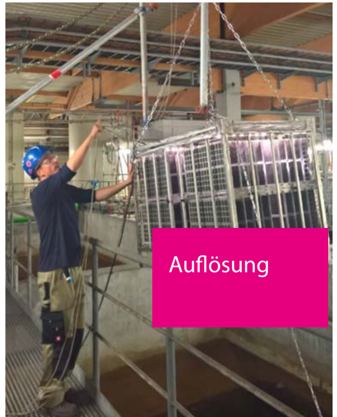
Fig. 2: Installation of catalystmodule at make-up water supply of power plant
