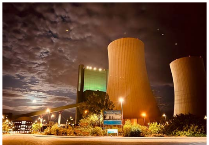
Fig. 3: Power plant of SaaleEnergie in Schkopau/Germany
