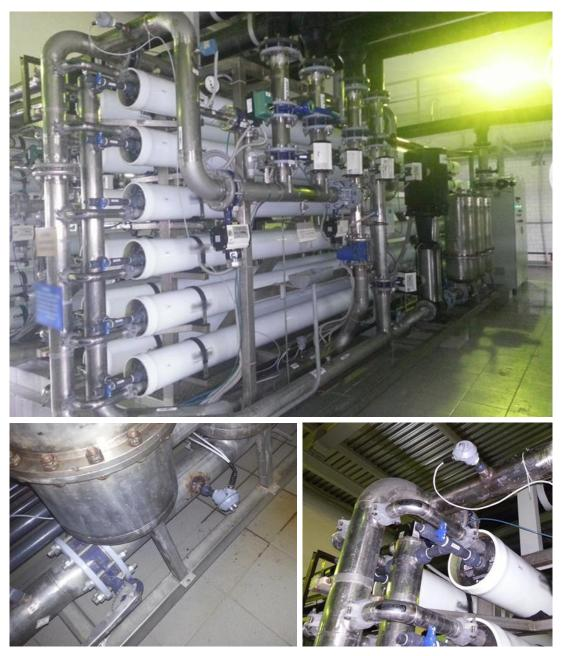
Figure 3: Overview of RO system (on the top), ALVIM Sensor installed before RO (on the bottom, left), ALVIM Sensor installed in the concentrate line (on the bottom, right)
