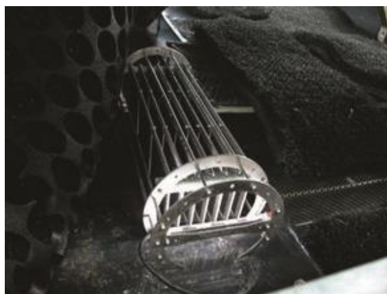
Fig. 4. MOLLIK-module installed at cooling basn (Körner et al., 2015)
